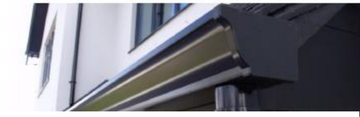
Extruded aluminum guttering
