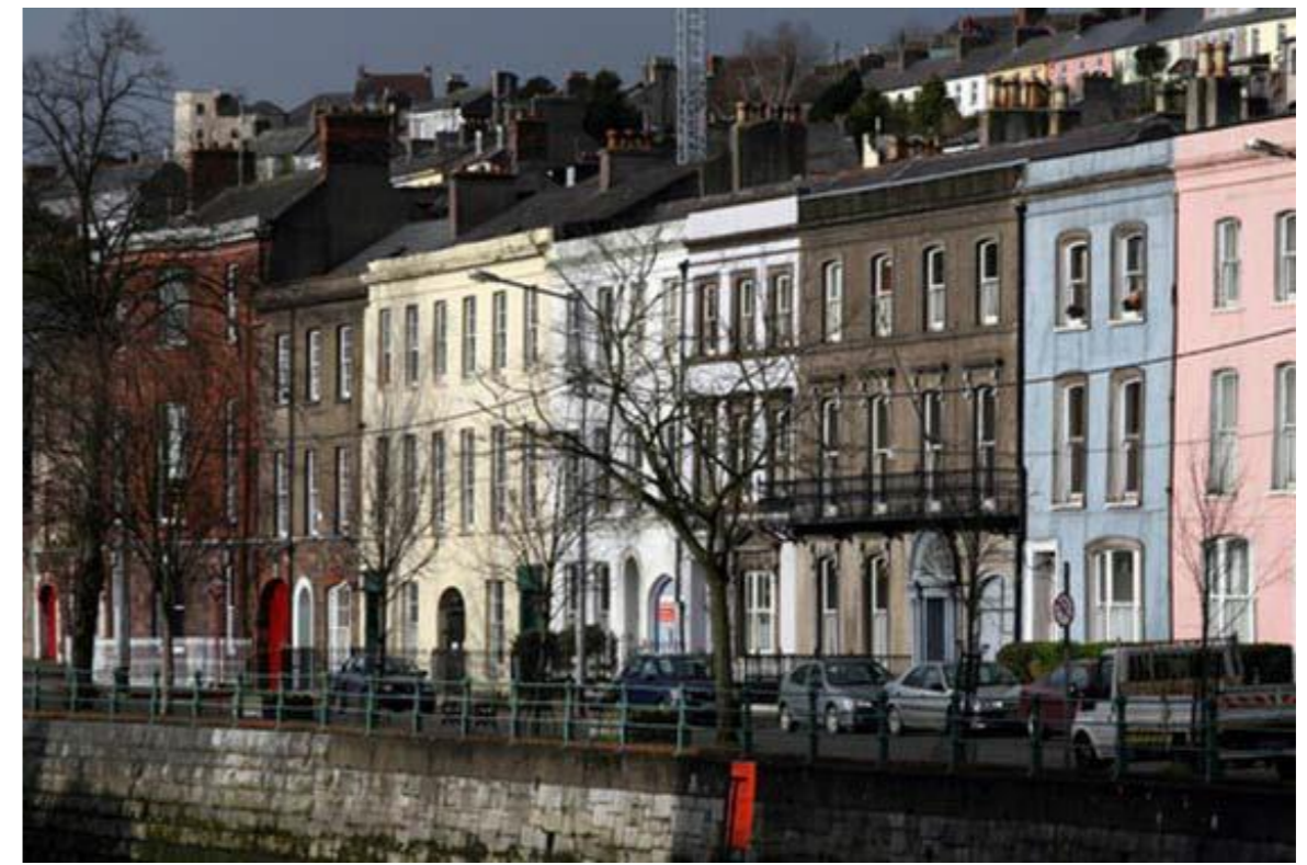
Plaster, brick &.slate finish to streetscape.
