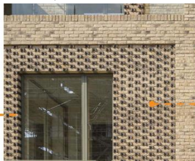
Recessed panel detail to front elevation with feature header to selected areas
