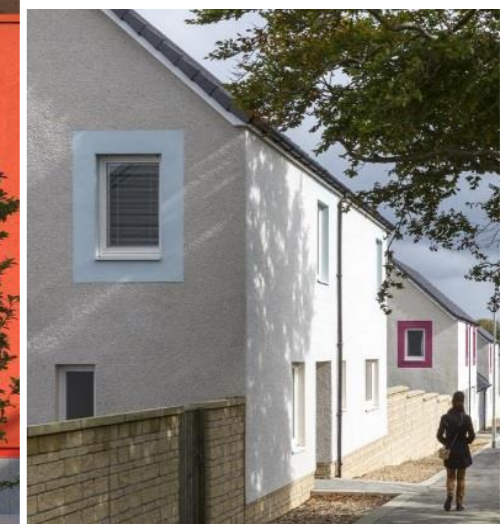
Render Detail around window openings
