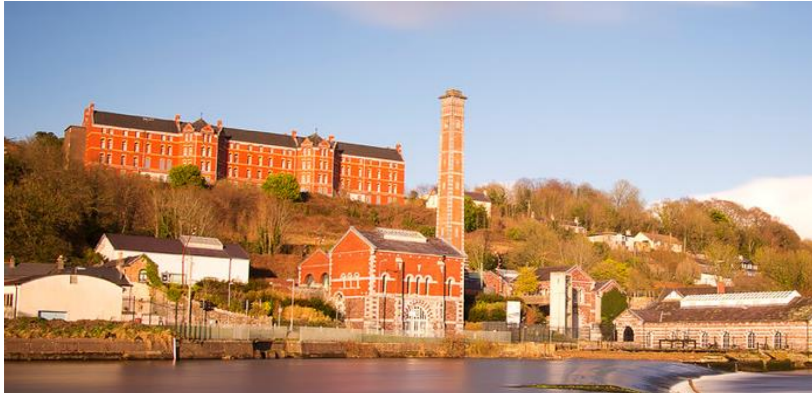
Red Brick Use at St. Kevin's Hospital and Old Cork Waterworks Building below the site.
