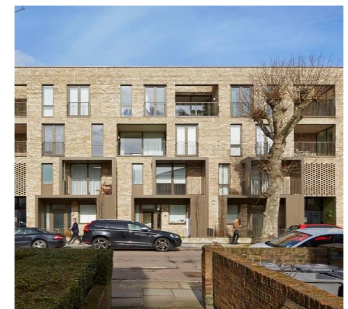
Buff Brick Reference Images . Ely Court, South Kilburn by Alison Brooks Architects.
