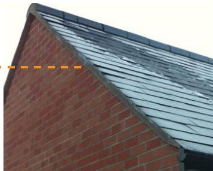
Flush gable brickwork to fibre cement slate soffit
