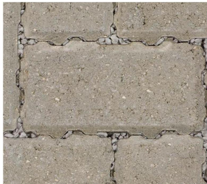
Car Parking Paving - Permeable PCC Pavers
