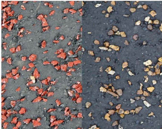
Shared Surface - Hot Rolled Asphalt with Colour Chip
