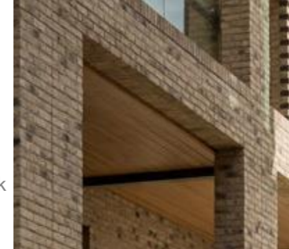
Returning brick soffit to balcony changing to hardwood timber cladding to soffit
