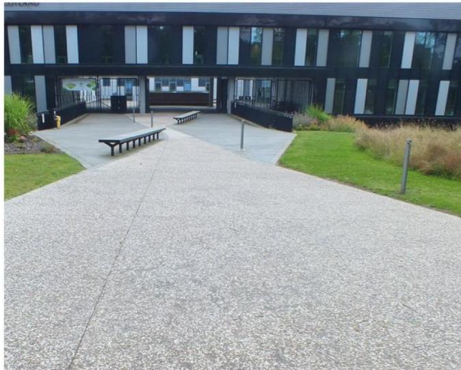
Secondary Paving - Exposed Aggregate cast in-situ concrete
