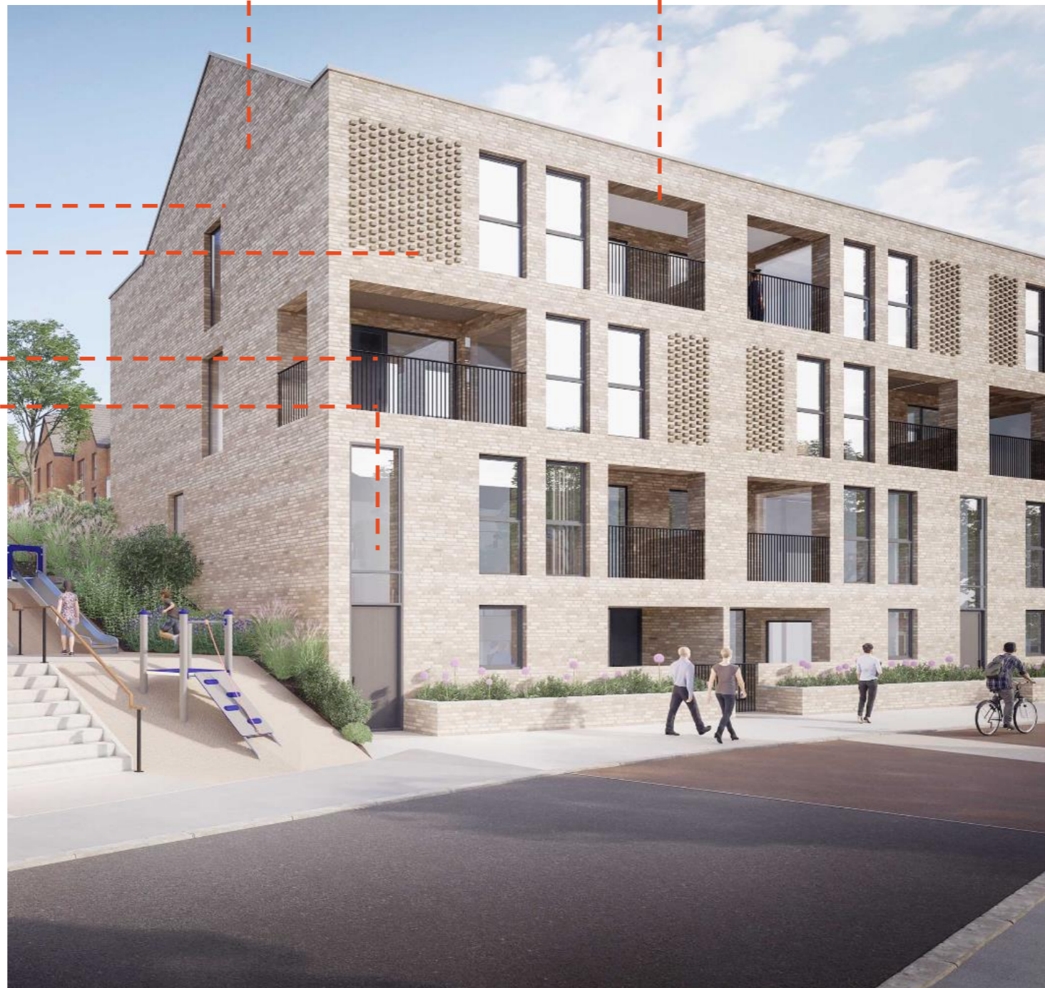
Returning brick soffit to balcony changing to hardwood timber cladding to soffit
