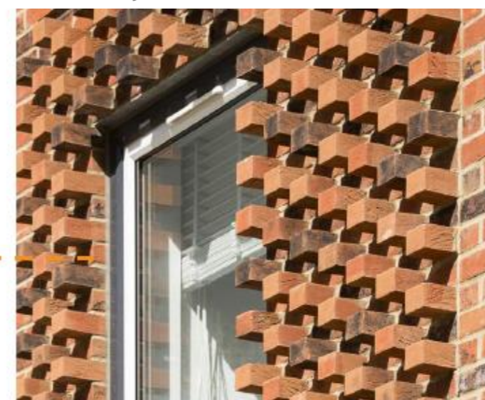
Feature header detail to selected areas with brick window reveal
