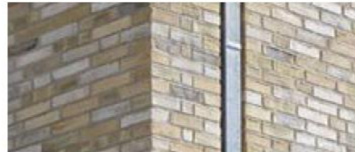
Extruded aluminum recessed downpipe detail
