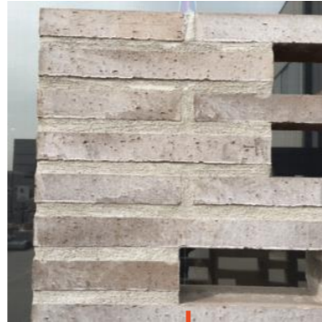
Flush pointed brickwork with Light mortar
